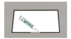
Close to the edge of a circumferential Pactanraupe. Apply consistently without interruption to prevent a later penetration of moisture downwards.
